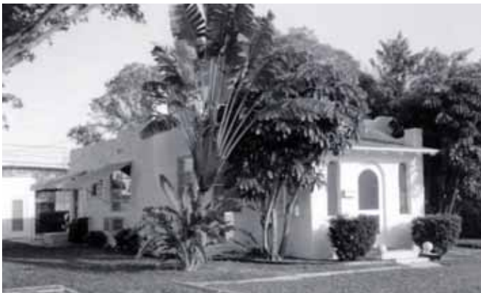
Figure 3. 1925 Mission Style House Located at 823 SE 4th Avenue
