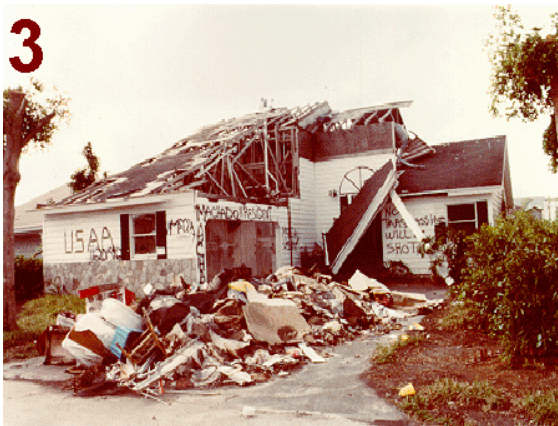
MAJOR DAMAGE UNINHABITABLE
