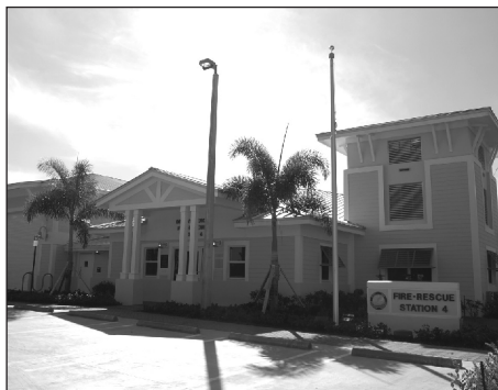
Newly rebuilt Fire Station 4
