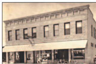
The Cathcart Building, built in 1912 will be featured in the "Mid-Century Signs of Commerce" exhibit.
