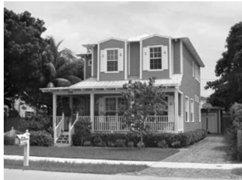
An example of appropriate infill construction in the Del-Ida Park Historic District
