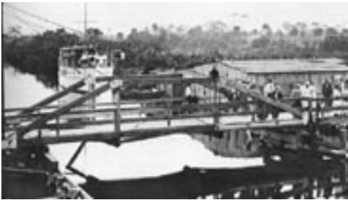
Circa-1910 photograph of the original bridge over the East Coast Canal (Intracoastal Waterway)
