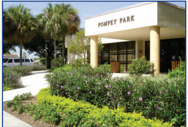
Renovations to the Pompey Park Community Center include a new entrance on the east side.
