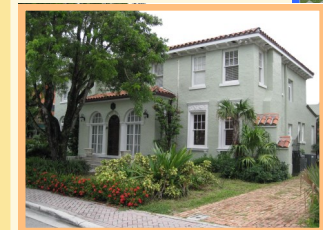
238 NE 1st Avenue, Banker's Row
